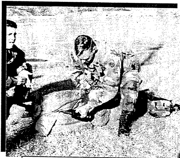
Use of sandbags to zero the bore light in the field.
